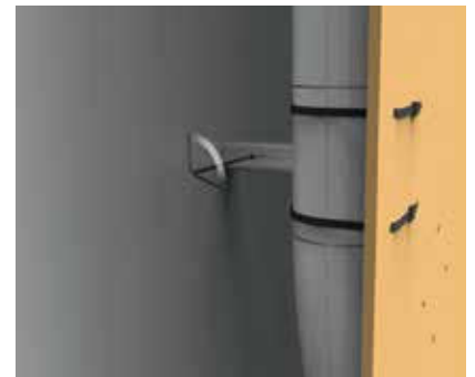
6. Detail of the wall pins fixing.
