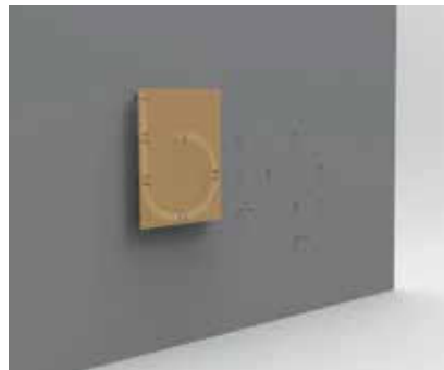
4. Attachment of letter b on wall pins.
